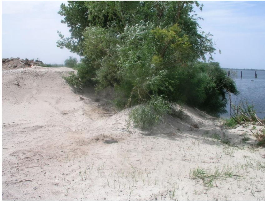
Fig. 4. Reworking of the coastal slope of the cooling pond dam from the side of the Kakhovka Reservoir (photo 2010)
