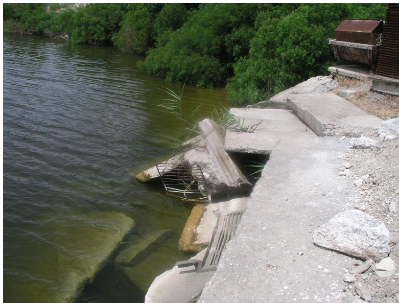
Fig. 3. Destruction of the slope fastening at the pumping station supplying water to the cooling towers (photo 2010)
