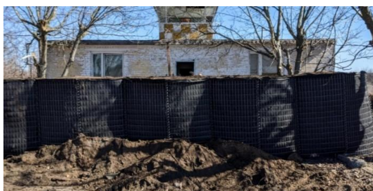
Fig. 2. Axial gabion ( https://cutt.ly/me6IYClq )
