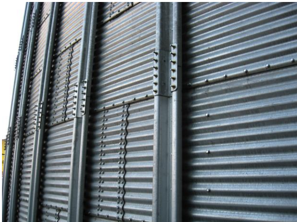
Fig. 1. Packets of sheets from thin-walled galvanized profiles for steel silo capacitive structures
