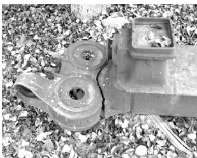
Fig. 5. General view of the fractured beam
