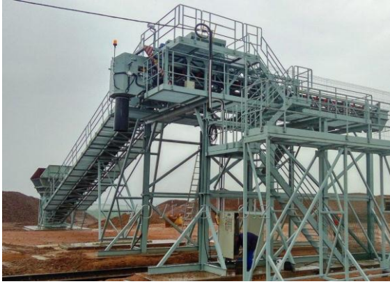
Fig. 2. Automated system of the dose loading of broken stone in cars
