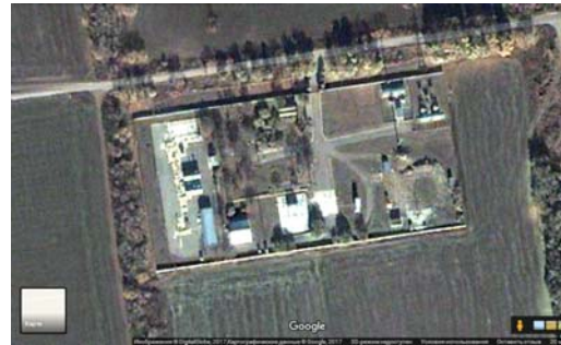
Fig. 2. Ammonia pump station
